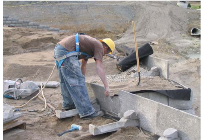
Attaching Lock and Load™ face 'stone' to counterfort
