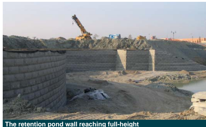
The retention pond wall reaching full-height
