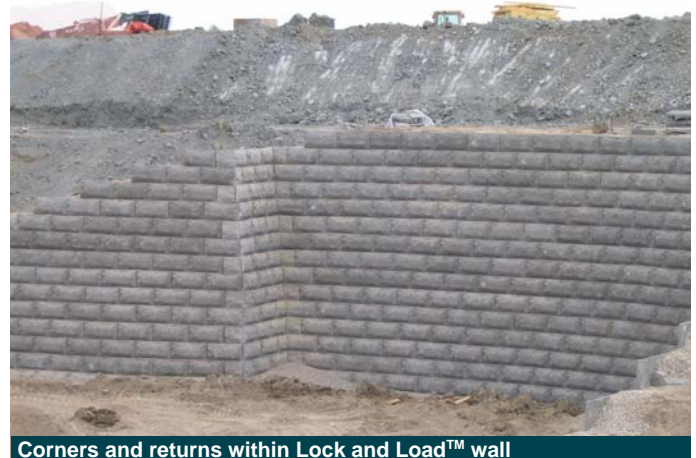
Corners and returns within Lock and Load™ wall
