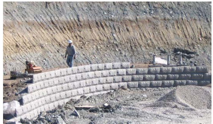
Backfill compacted onto soil reinforcement geogrids
