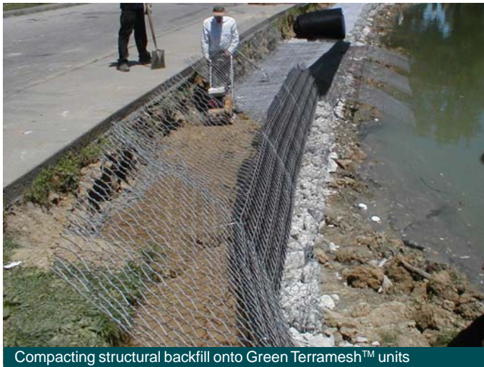
Compacting structural backfill onto Green Terramesh™ units
