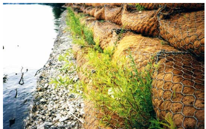
Live planting installed between Envirolog™ layers
