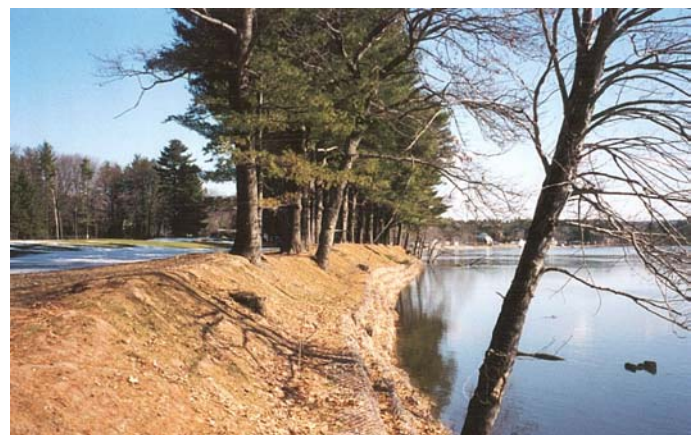
Completed structure, awaiting live planting
