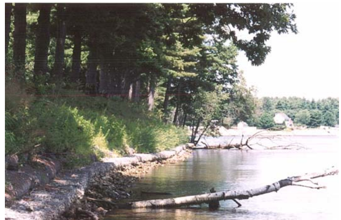
Vegetation establishing in completed structure
