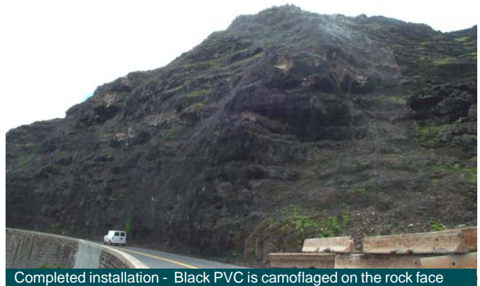
Completed installation - Black PVC is camouflaged on the rock face
