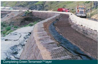
The coir net has 75% open area which allows intimate contact between the hydoseed and the quality topsoil, increasing the potential for seed germination.
