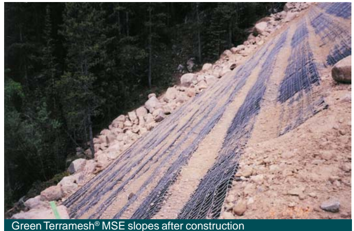
Green Terramesh® MSE slopes after construction
