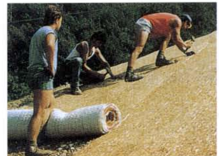
Installation of Biomac® along a slope to protect against erosion.
