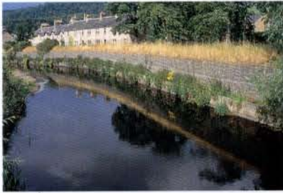
River bank protections with gabions manufactured with double twisted steel wire mesh. Gabion units are filled with stones integrated with live plants using bio-engineering techniques.
