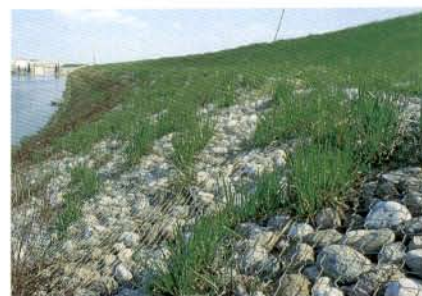
Bank Protections with Reno mattresses manufactured with double twisted wire mesh. Reno mattresses are used to cover large surfaces. They can be combined with live plants, sealed with soil or vegetative pockets.
