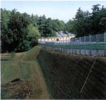
Reinforced Soil slopes with Green Terramesh® .
