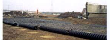
Reinforcement of embankment on piled foundations with high strength polyester Paralink.
