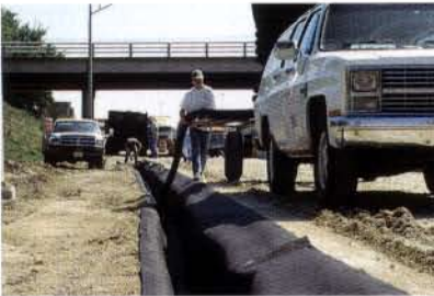
Filtration, separation, drainage for earthworks with MacTex® Non Woven geotextiles.
