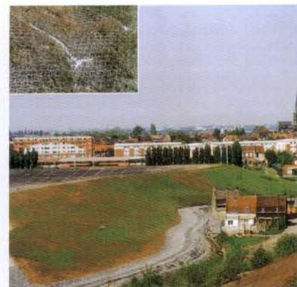
Vegetative linings with Geomac® mattress in double twisted steel wire mesh, internally lined with a geotextile.
