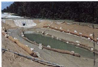
Protection works of a stormwater management area using Waterlogs.
