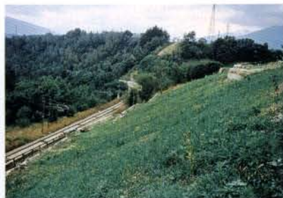
Macmat®R for bank and slope erosion protection. MacMat®-R is a geocomposite TRM reinforced with double twisted steel wire mesh.
