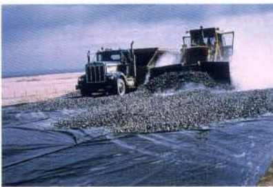
MacTex® Woven geotextiles for soil separation and erosion control.
