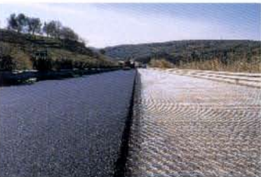
Paving reinforcement with Road Mesh® , a double twisted wire mesh reinforced with steel rods across the weave direction.
