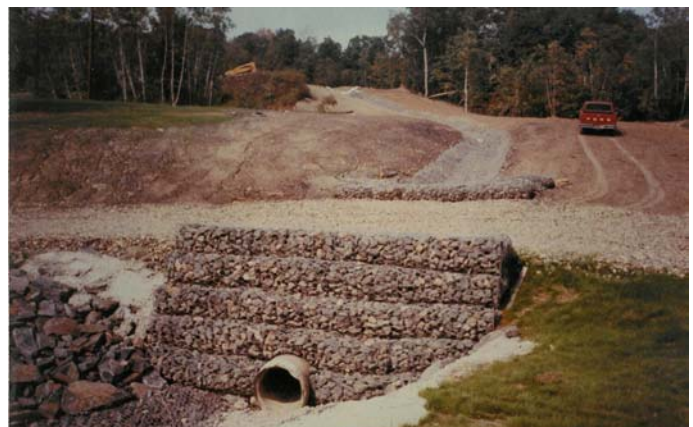
Gabion culvert retaining structure supporting accessway
