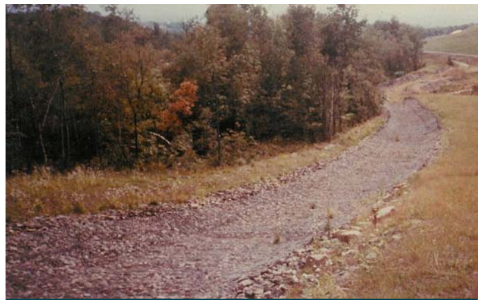
12" thick gabions protecting downchute
