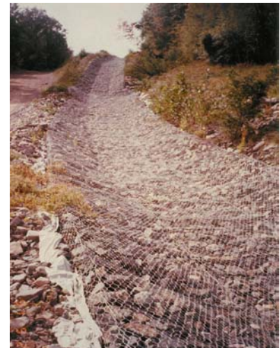
12" thick gabions used on downchutes
