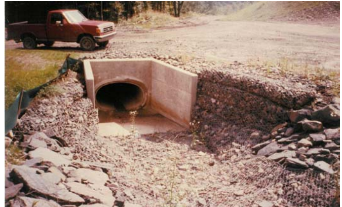
Gabions and Reno mattresses protecting culvert
