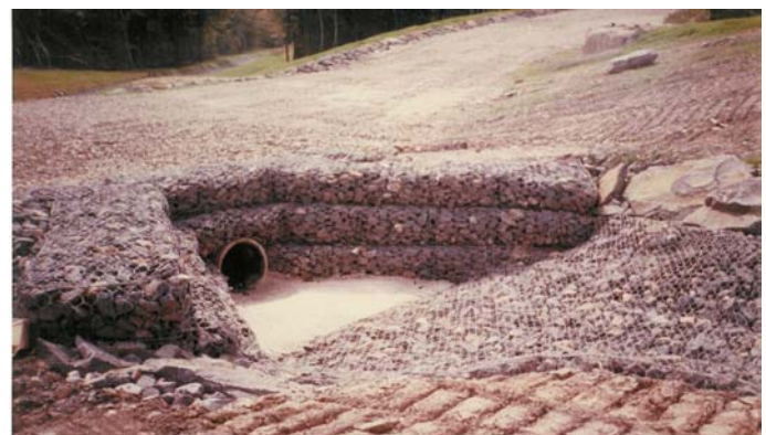
Gabion culvert protection
