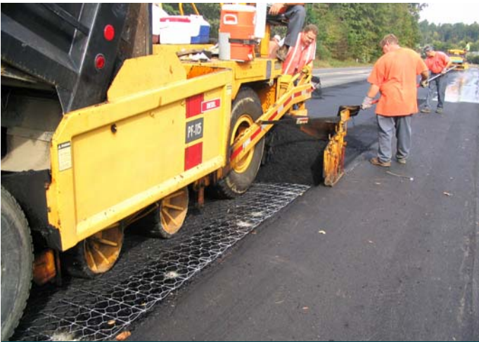
Placing asphalt using wheeled paver
