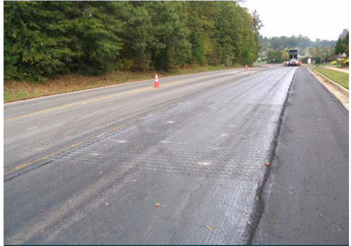
Fixed Road Mesh™ ready to receive wearing course
