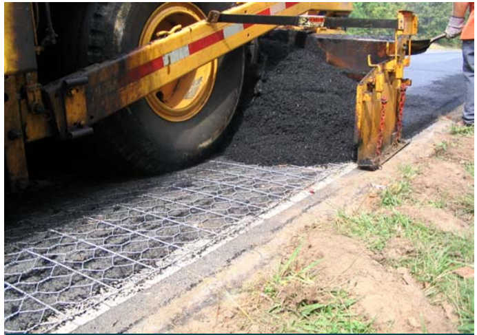
Placing new wearing course
