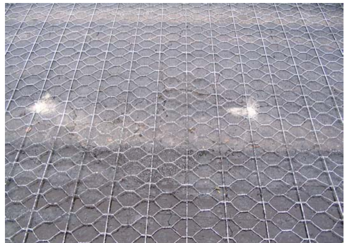
Road Mesh™ secured using Hilti™ fixings
