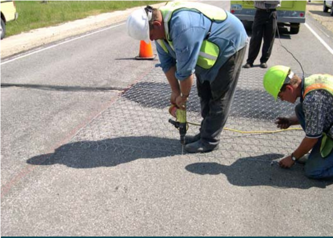
Securing Road Mesh™
