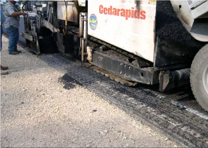
Placing asphalt wearing course
