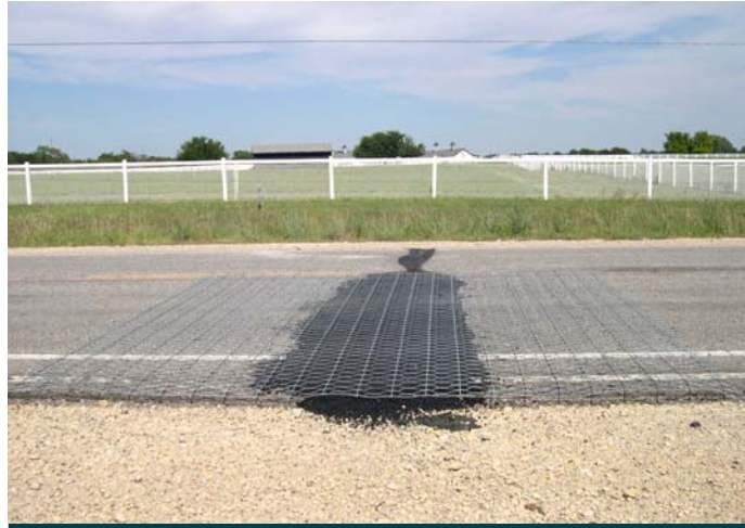
Road Mesh™ ready to receive wearing course
