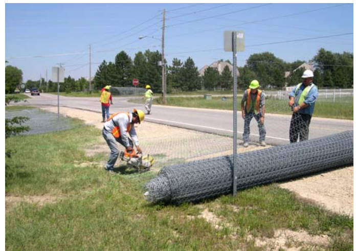
Cutting Road Mesh™ to correct lengths
