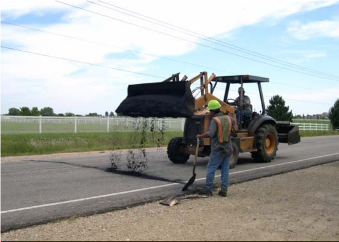
Filling crack with asphalt
