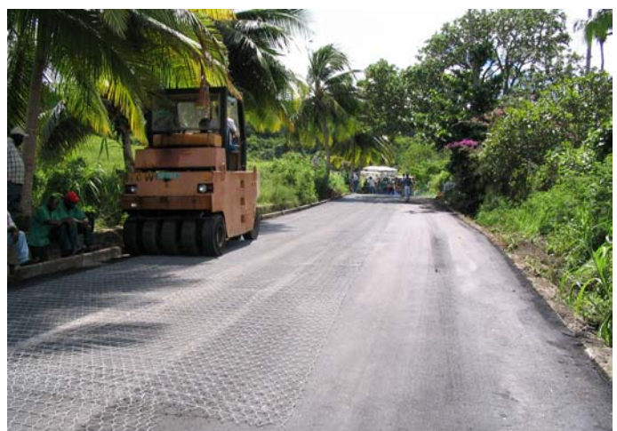
Deploying and rolling Road Mesh™ flat
