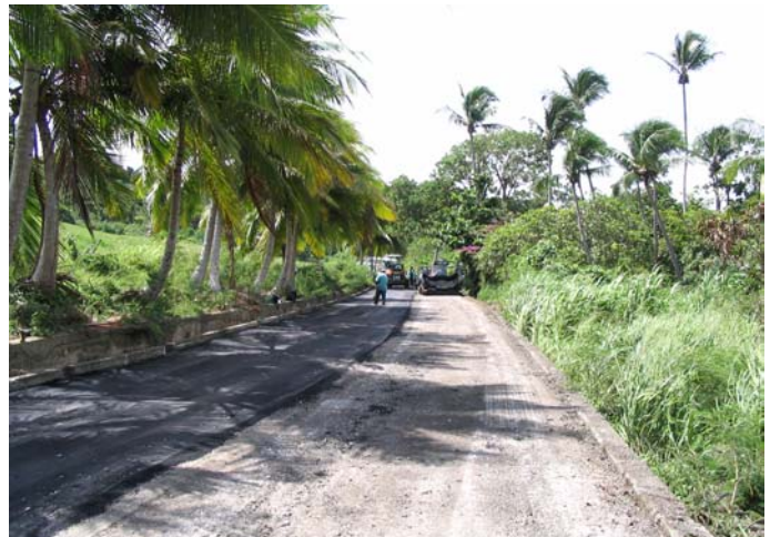
Placing 0.5" 'scratch' coat
