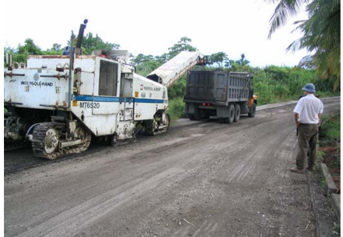
Milling existing pavement by 1.5"
