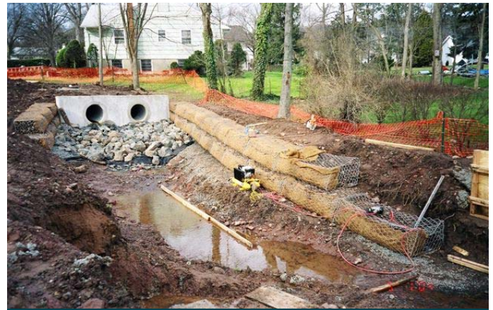
Green Gabions™ being filled with rock and topsoil
