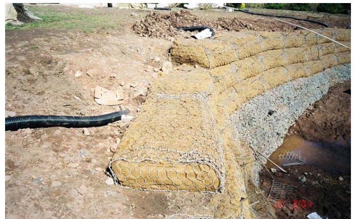
Completed Green Gabions™ awaiting live planting
