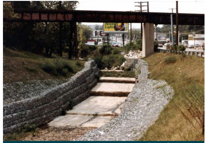
View upstream towards drop-structures
