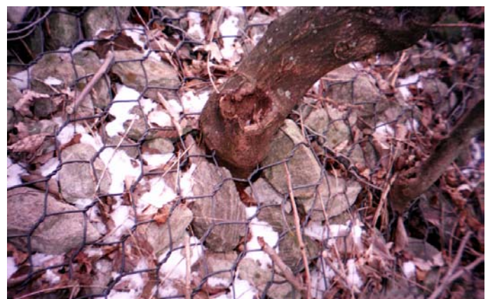
Vegetation through gabion
