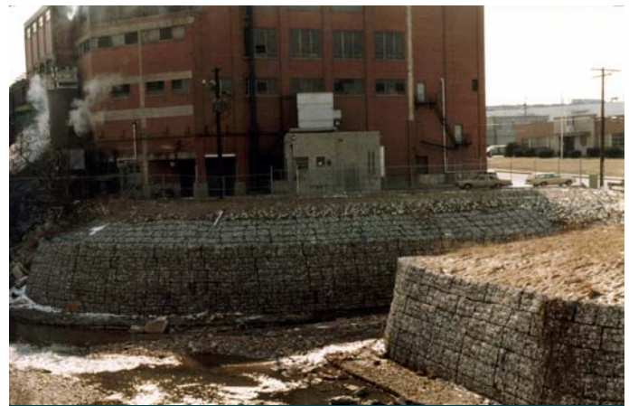
View of completed structure
