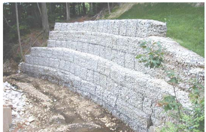
Gabion retaining wall and Reno Mattress channel lining
