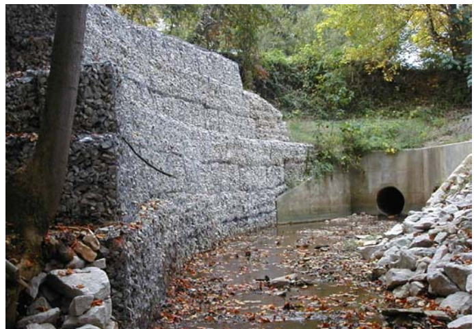
Completed gabion structure showing 'return'
