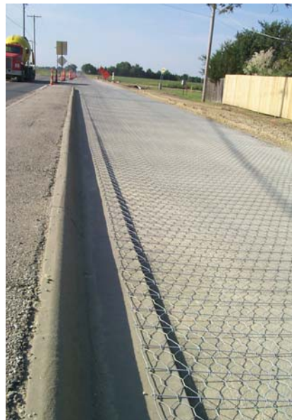
Road Mesh™ unrolled into position
