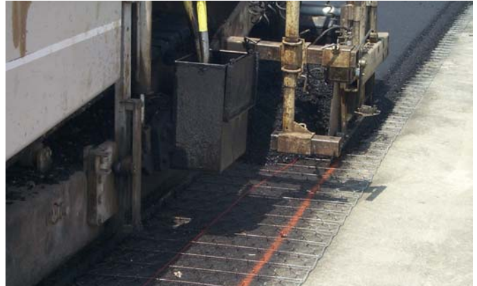
Asphalt courses applied directly onto Road Mesh™
