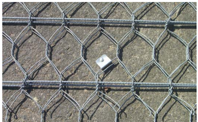
Detail of Hilti fixing at junction between two rolls of Road Mesh™
