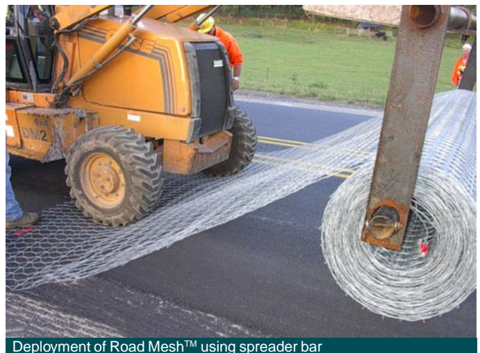
Deployment of Road Mesh™ using spreader bar
