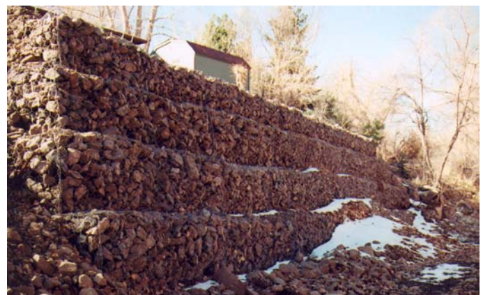
Completed gabion structure at downstream end
