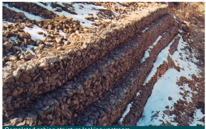
Completed gabion structure looking upstream
