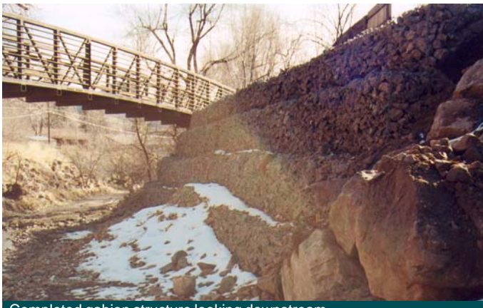
Completed gabion structure looking downstream
