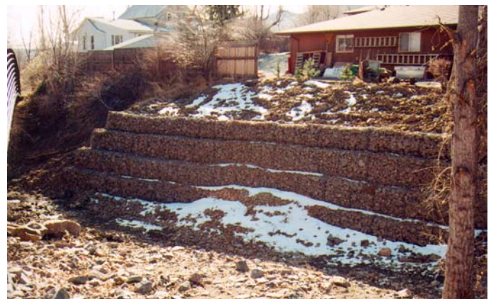
Completed gabion structure
