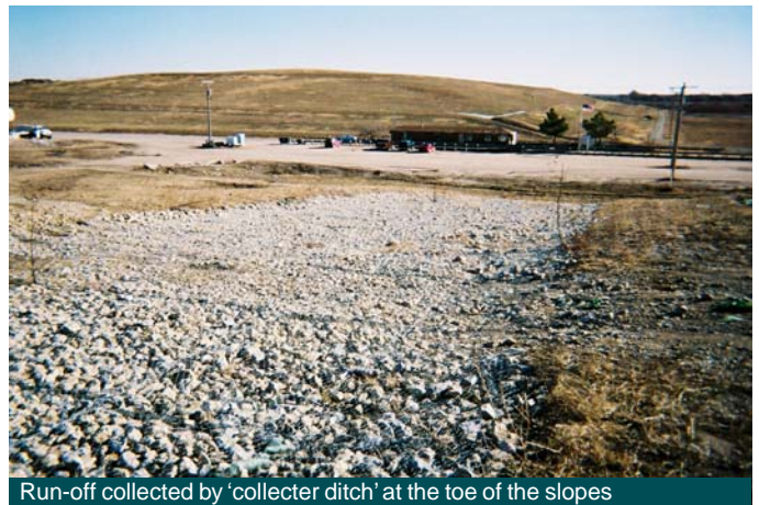
Run-off collected by 'collector ditch' at the toe of the slopes
