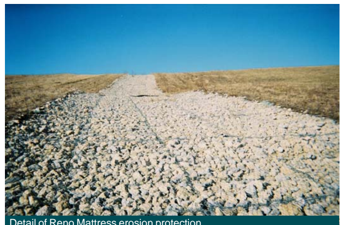
Detail of Reno Mattress erosion protection
