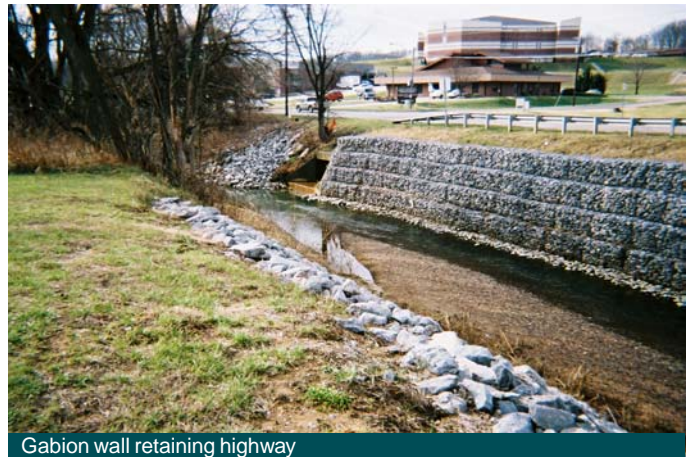
Gabion wall retaining highway
