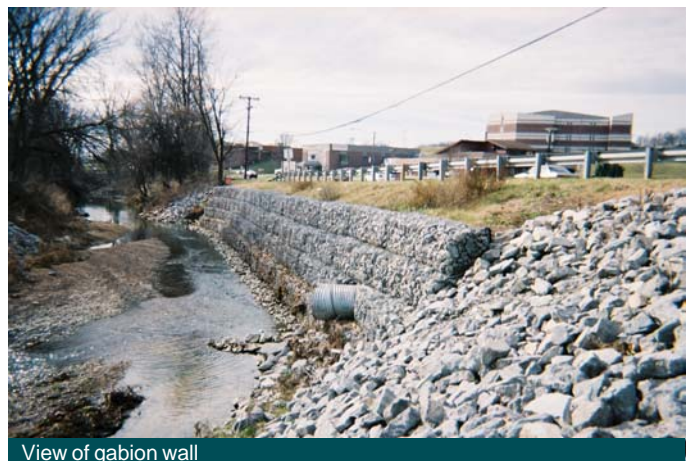
View of gabion wall
